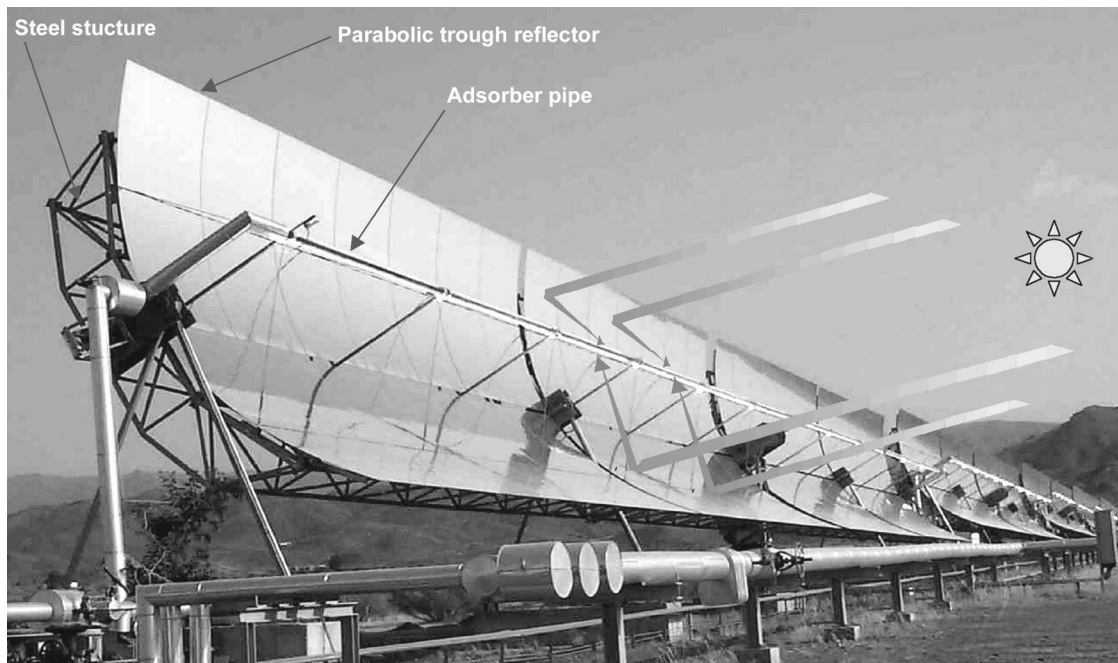
Fig. 3 Parabolic trough collector (source: PSA)
