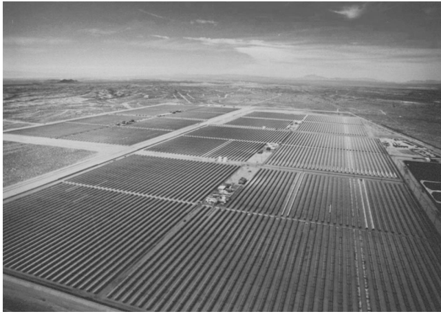
Fig. 2 SEGS III–SEGS VII solar plants at Kramer Junction, CA. The large fields with rows of parabolic trough collectors are readily apparent. The five 30-MWe power plants can be observed near the center of each solar field.
