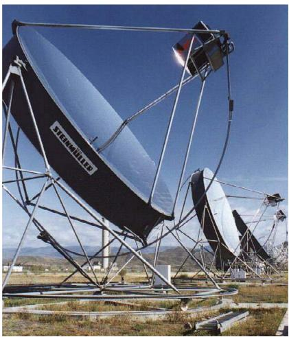
Figure 3.10 New SBP 10kW Dish-Stirling System at the Plataforma Solar de Almeria, Spain
