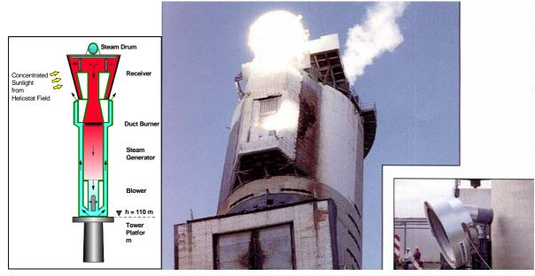
Figure 3.6 Schematics of Commercial Size PHOEBUS Receiver and View of 2.5MWt TSA Pilot Receiver operating at the Plataforma Solar de Almeria.
