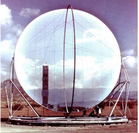
Figure 3.7 ASM-150 advanced stretched-membrane heliostat developed for PHOEBUS
