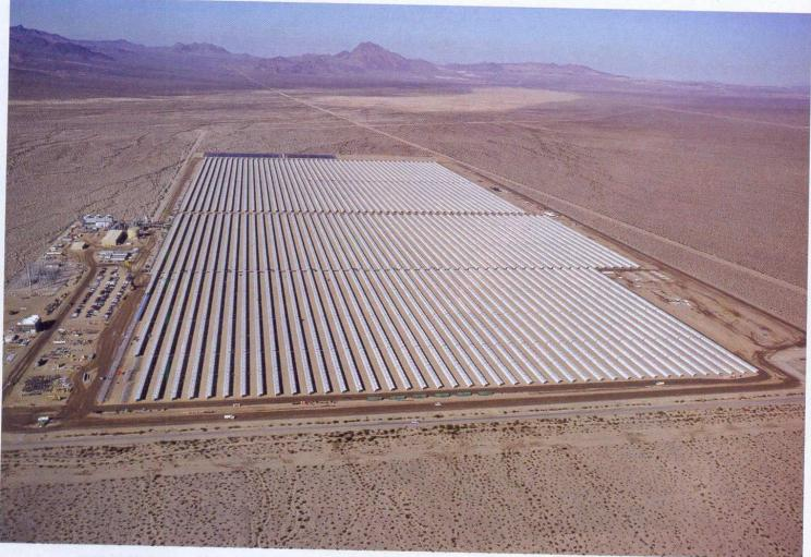
2. Closed-loop system. The heated heat-transfer fluid is circulated to a steam generator to produce superheated steam in a conventional steam turbine cycle. Courtesy: Acciona Solar Power
