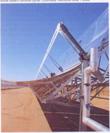
**3. Focused energy.** Schott AG supplied the 19,300 solar receiver tubes, each over 12 feet long, that capture the focused energy of the sun to heat a heat-transfer fluid that circulates through the receivers. *Courtesy: Acciona Solar Power*
