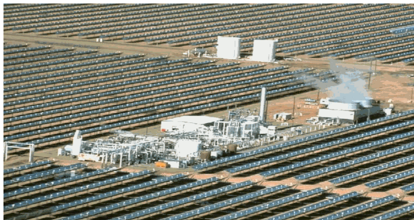
Figure 3 — Solar Trough Generating Plant
