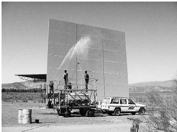
Fig. 8. A Spanish designed heliostat, of the type to be used in the PS10 tower project, being cleaned.
