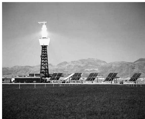
Fig. 7. The Solar Two central receiver plant in Barstow, California. This plant is now shut down but the next is under development for Spain as Solar Tres.
