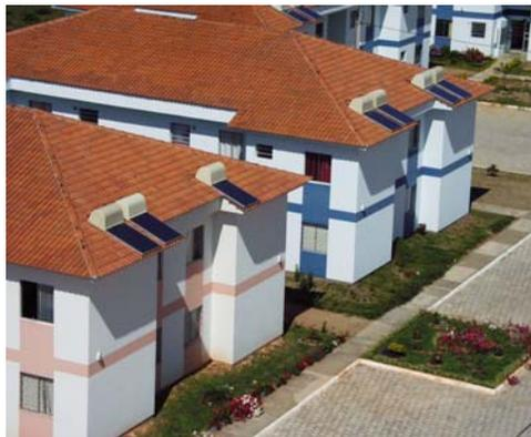
Figure 2. Compact solar domestic hot-water systems on the roof of the buildings
