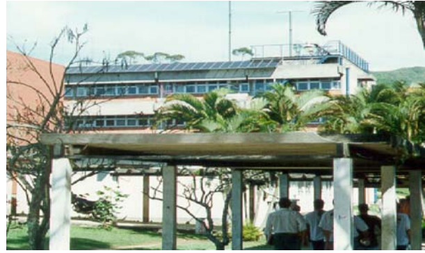
Fig. 1: 2 kWp a-Si:H grid-connected BIPV installation in Florianopolis, SC, Brazil
