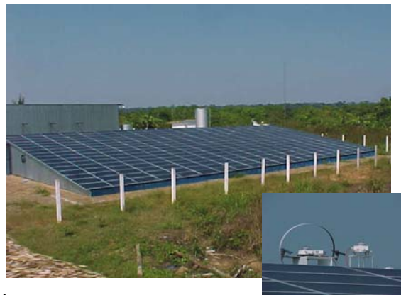
Fig. 2: Hybrid Diesel/PV installation in the Amazon, with a fully monitored, north-facing 20kWp PV system at latitude tilt (10°), and Diesel thermal plant in the background.
