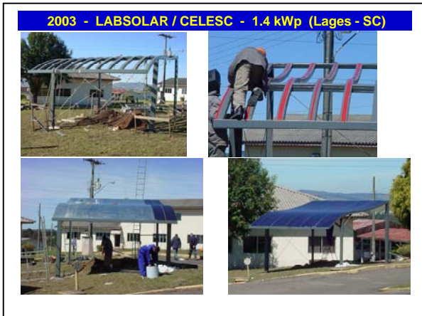
Fig.4: Lages – SC; one of the three BIPV systems installed in a joint project with the local electricity utility CELESC to monitor the performance and showcase grid-connected PV. The PV system uses flexible PV laminates which are field-applied onto a curved surface.
