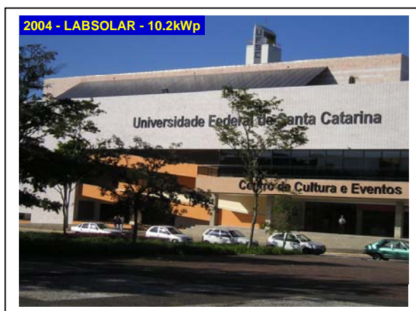
Fig.3: View of the University’s theatre BIPV system. The 10.2kWp installation showcases the PV technology to a widespread audience.
