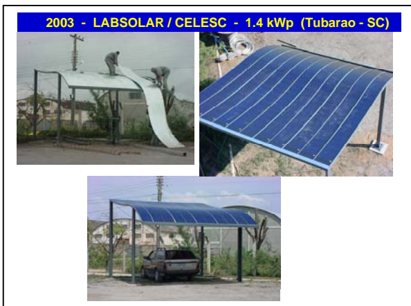
Fig.5: Tubarao – SC; one of the three BIPV systems installed in a joint project with the local electricity utility CELESC to monitor the performance and showcase grid-connected PV. The curved surface was designed to demonstrate the potential of PV laminates as a building element to architects and builders.
