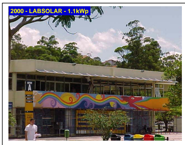
Fig.2: View of the University’s student guild building and its BIPV system. Disseminating the concept of on-site solar generation to the future generations of decision-makers is part of LABSOLAR’s efforts in making PV a more widespread technology.
