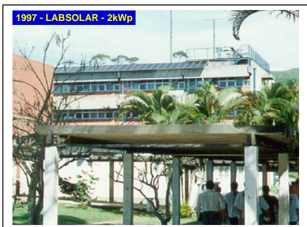
Fig.1: View of the first grid-connected BIPV system installed in Brazil. The 2kWp thin-film amorphous silicon installation uses opaque and semi-transparent glass-glass PV laminates, and is oriented towards true north at latitude tilt (27°).
