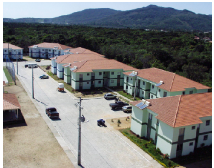
Fig. 2: Low-income family housing unit with installed compact solar water heating systems.
