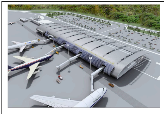
Figure 1: The new Florianopolis International Airport in Brazil is ideal for incorporating PV on both the brise-soleil surfaces and on the smoothly-curved and slightly-tilted roof-cover.
