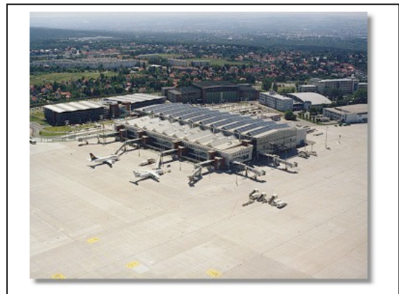
Figure 2: The Dresden International Airport in Germany, is well suited for PV integration on both passenger terminal and grounds (www.falconcrest.com).
