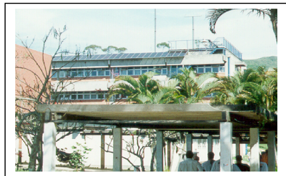
Figure 1: The 2kWp thin-film amorphous silicon BIPV system operating continuously since 1997 at the LABSOLAR building in Brazil.
