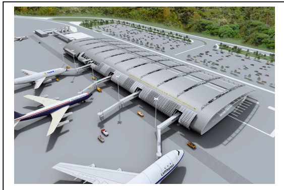
Figure 1: The new Florianopolis International Airport in Brazil is ideal for incorporating PV on both the brise-soleil surfaces and on the smoothly-curved and slightly-tilted roof-cover.
