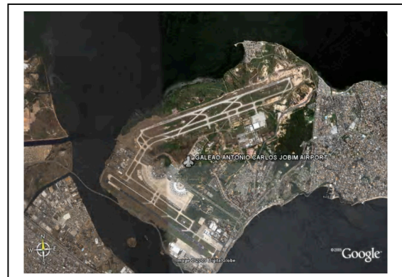
Figure 2: The Rio de Janeiro International Airport in Brazil, is well suited for PV integration on both passenger terminal and grounds.
