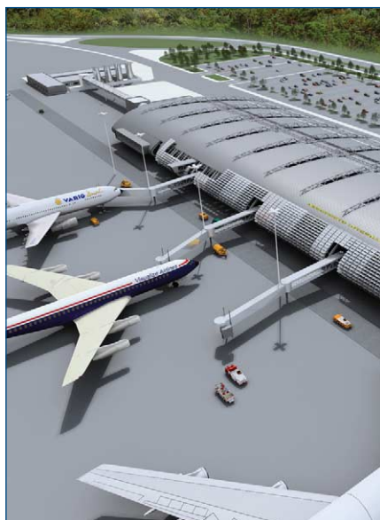
Figure 1: The project of the new Florianópolis International Airport in Brazil is ideal for incorporating PV on both the brise-soleil surfaces as well as on the smoothly-curved and slightly-tiled roof-cover
