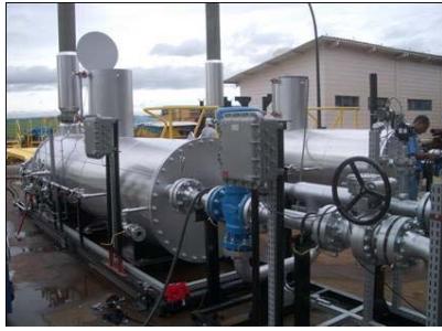
Figure 1: Actual water-bath heater.
